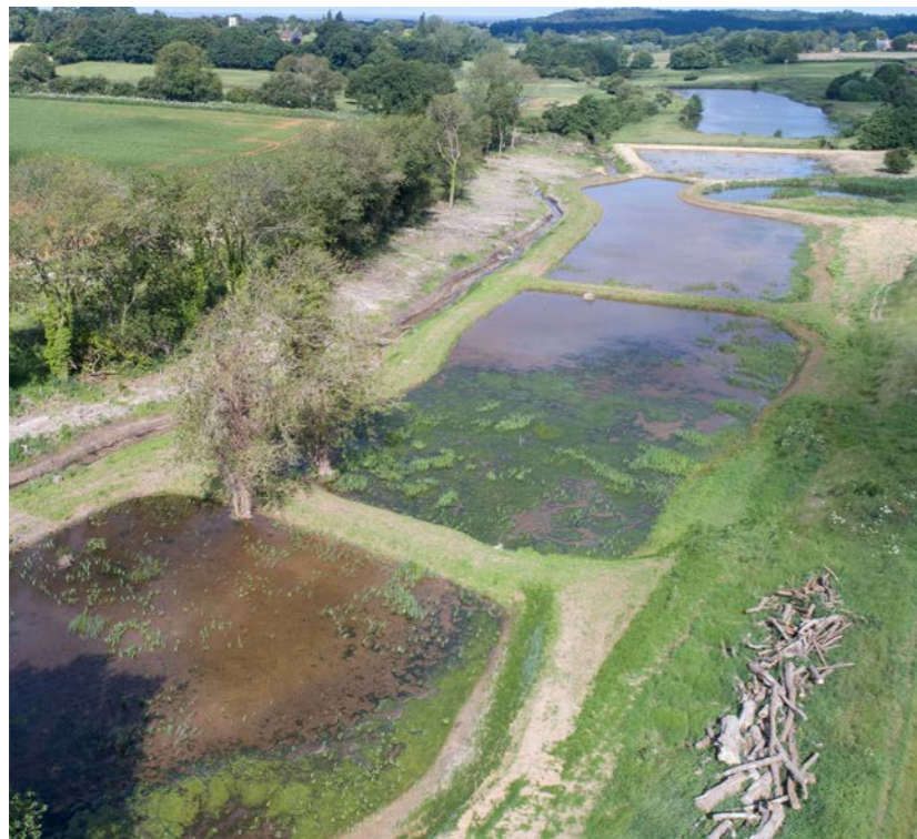
Example of wetland creation to improve water quality in the River Ingol at Ingoldisthorpe
