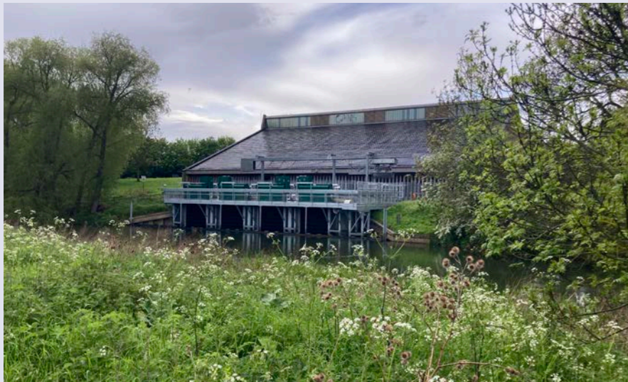
Example of a pumping station at Tinwell
