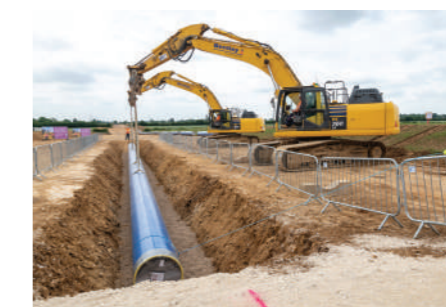
Example image of pipeline installation
