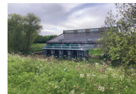
Example image of typical pumping station
