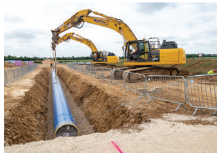
Example image of pipeline installation
