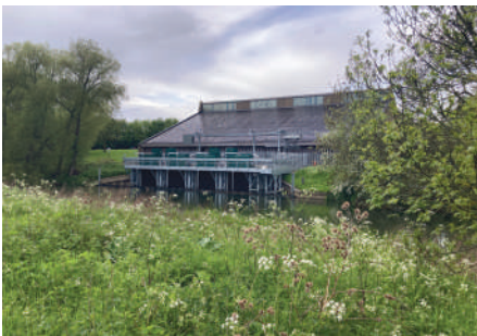
Example image of typical pumping station
