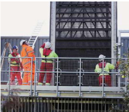
Example image of screen used at intake
